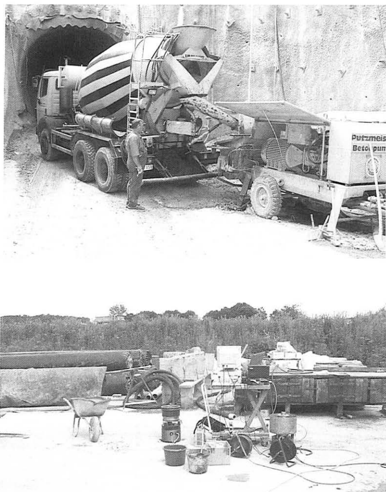
Figure VII.5 – Chantier de Pforzheim.
